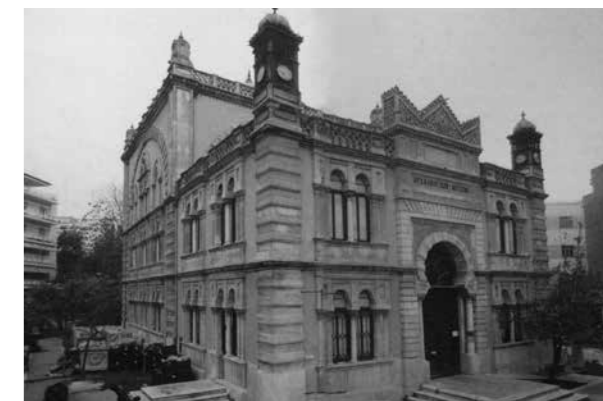
View of Yeni Mosque
